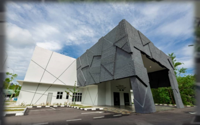
The front facade of the building (above) was designed after fracture pattern of the limestone karst wall by the side of the discovery centre.
